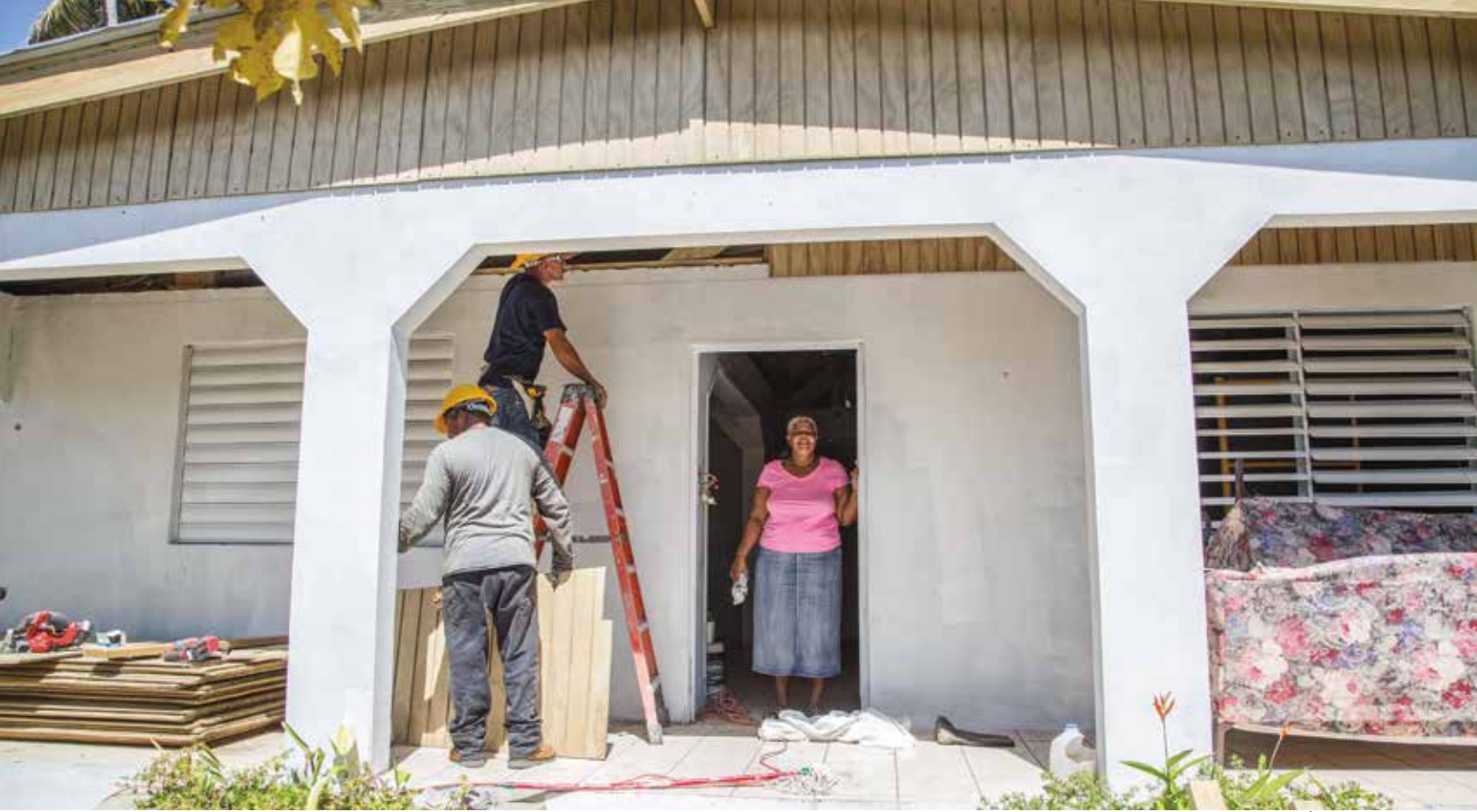
One of the houses rehabilitated in Loíza.
