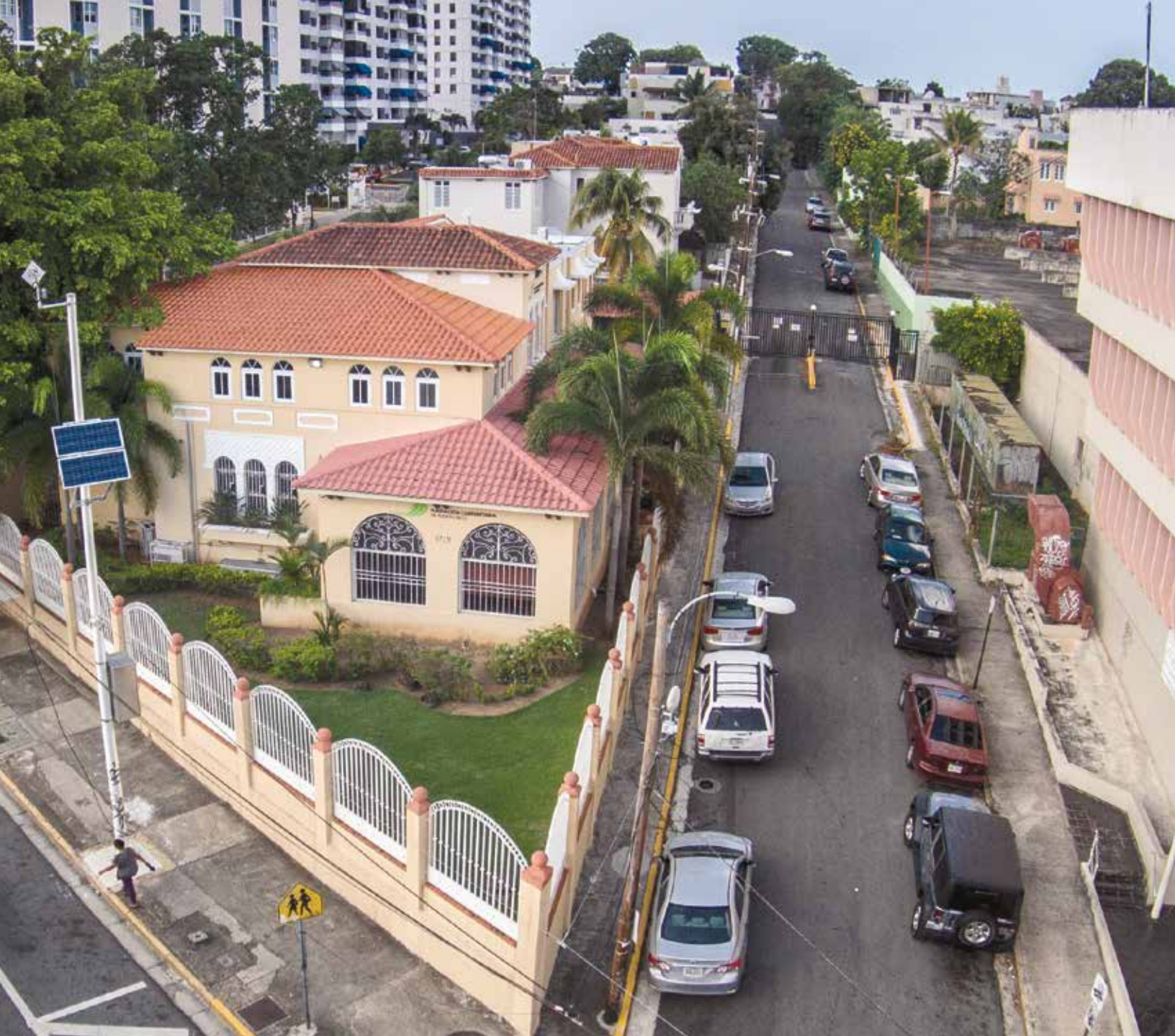
Puerto Rico Community Foundation main office in San Juan, Puerto Rico.
